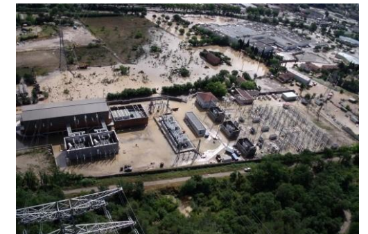
2010 floods : structures on stilts were not impacted
